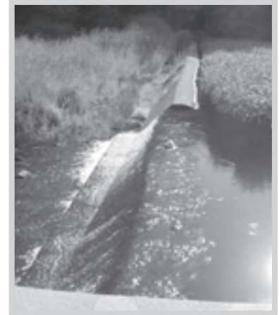
Photo: Segreganset River Dam, Dighton.
