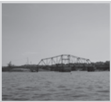
Photo: Historic Berkley-Dighton Bridge.
