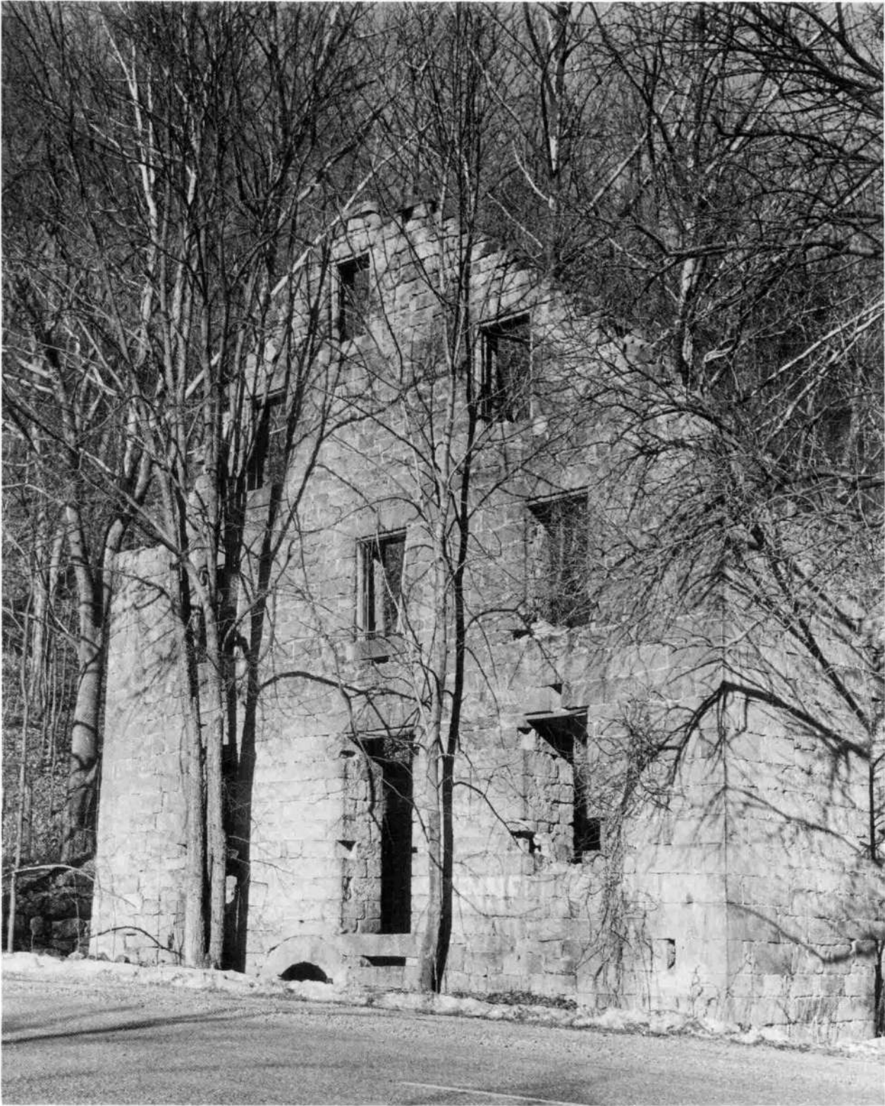
Standing on the north bank of the main stem at the site of the old settlement of Sprucevale is Hambleton's Mill, the last remaining structure of that former settlement.
