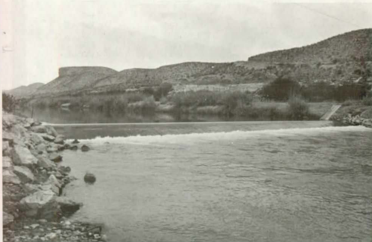
A five-foot weir at the Foster Ranch gaging station, immediately downstream from the Terrell-Val Verde County line.
