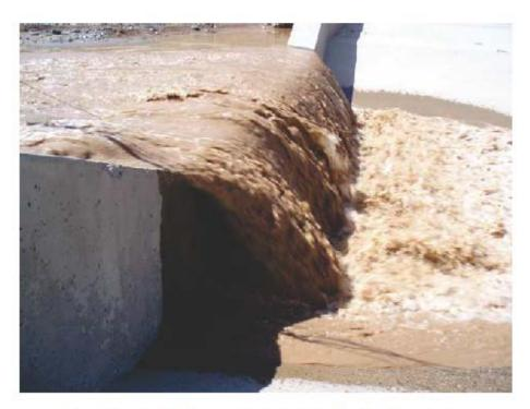
Figure 4: Aravaipa Fish Barrier that is Similar to the Blue River Barrier Design.
