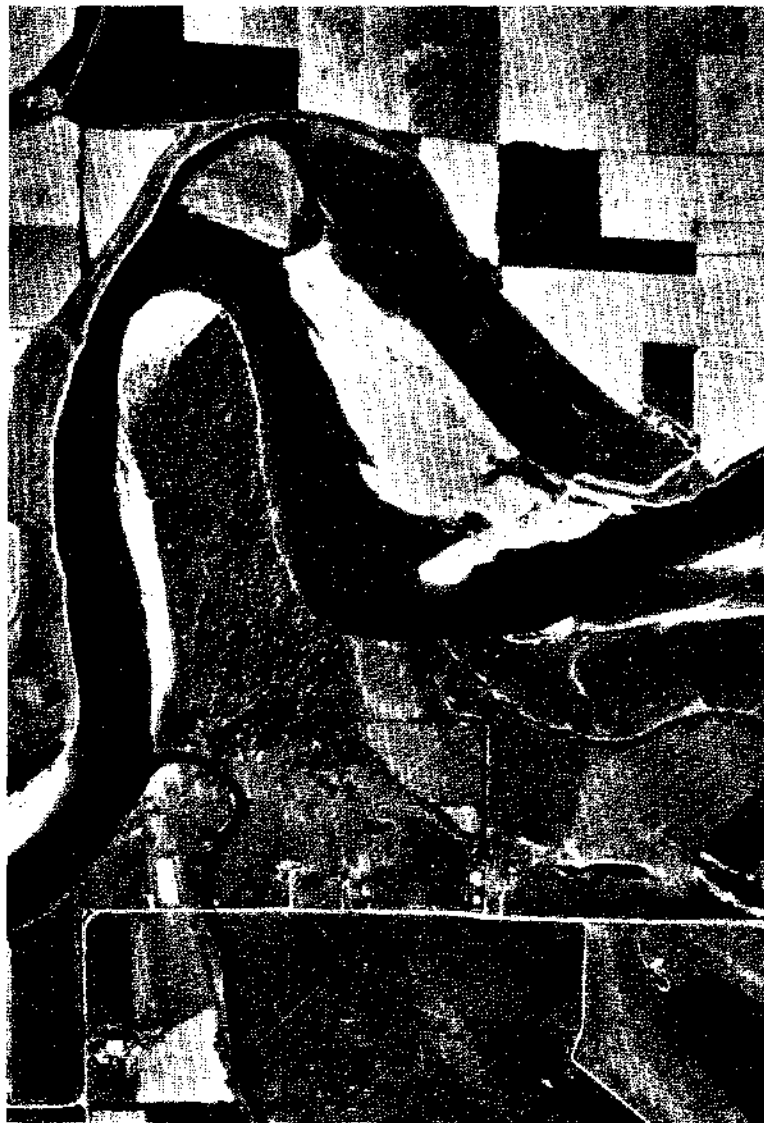
Photo 2 - The same oxbow thirty years later. In this 1971 picture the agricultural land has been totally eroded away. Note the new main channel, gravel bar and backwater created.
