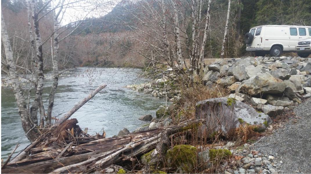
**Figure 26 - Example of rip rap that has been placed in the MF to protect the Middle Fork Road.**
