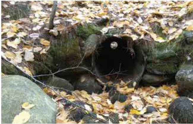
*Poorly or undersized culverts can create high water velocity, turbulence, and/or inadequate water depths within the culvert leading to migration barriers for fish and other aquatic species. They also restrict natural stream flows, particularly during floods.*
