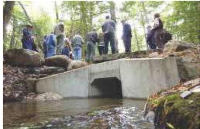
*Replacing old pipe culverts with new bottomless, three-sided culverts helps provide passage for fish and other aquatic species. Such projects often necessitate the efforts of multiple partners to accomplish, such as here with Trout Unlimited's involvement with a Gulf Brook culvert in Pepperell, MA. Photo: NRWA Archives.*
