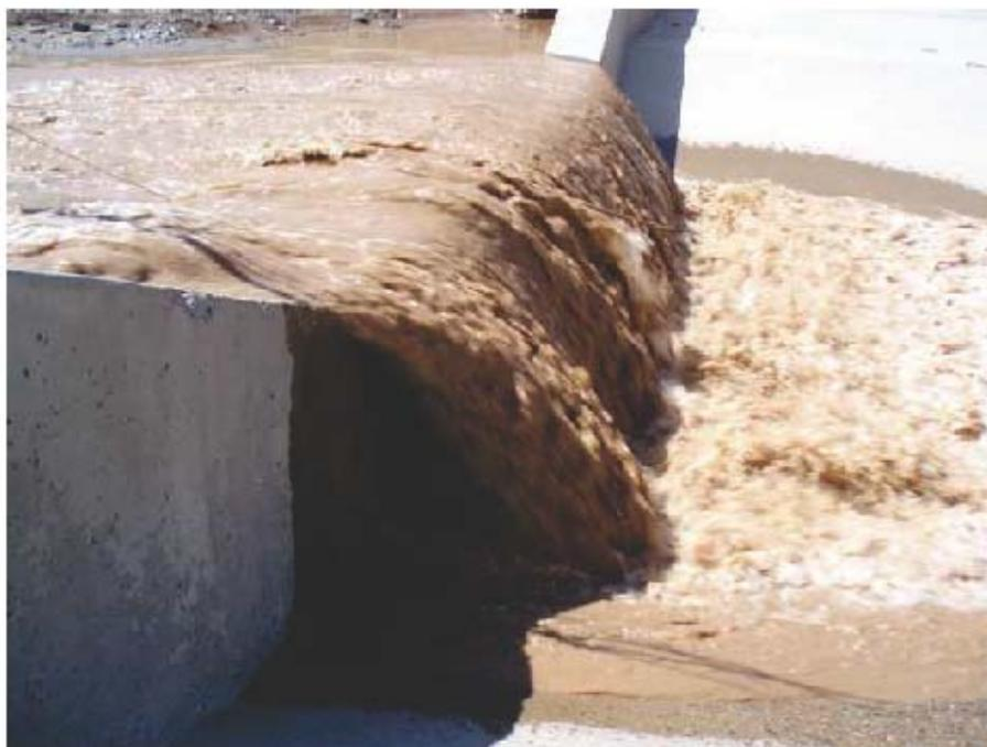
**Figure 4: Aravaipa Fish Barrier that is Similar to the Blue River Barrier Design.**
