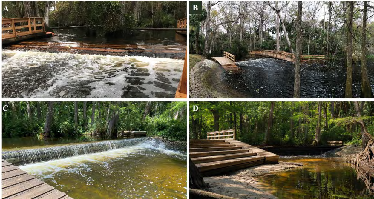
Figure 4.17. (A) Downstream and (B) upstream views of Lainhart Dam and downstream views of Masten Dam during (C) typical and (D) low river stages after the 2017 renovations. (Photos A, B, and D by SFWMD; photo C by A. Arrington).
