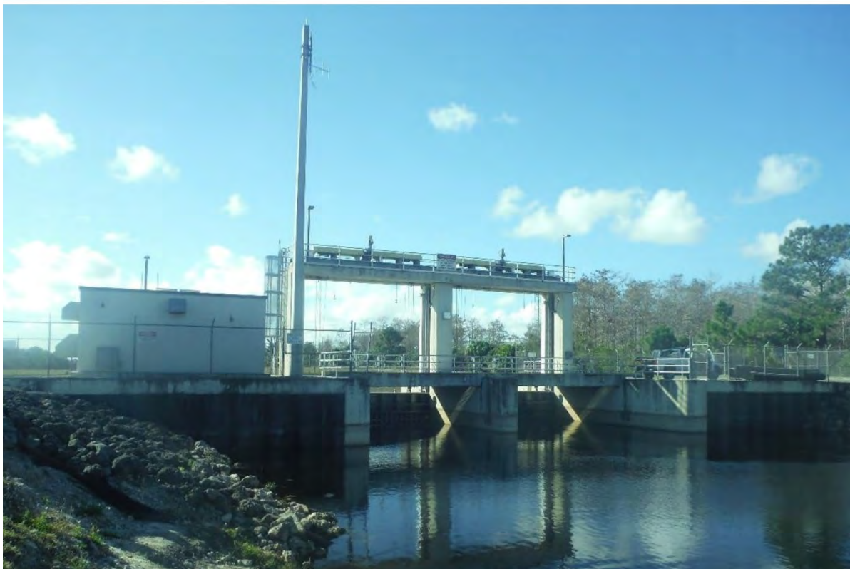
Figure S4.4. Upstream (top) and downstream (bottom) views of the G-160 spillway.
