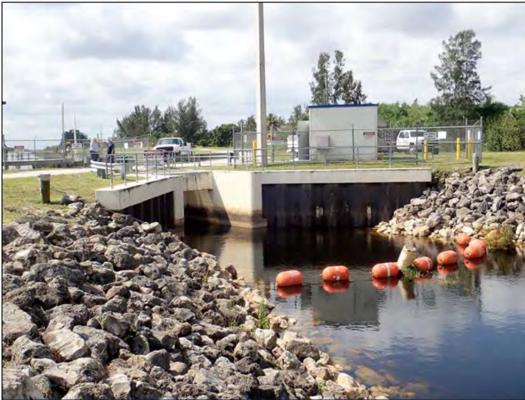
Figure S4.2: G-92 upstream and downstream view.
