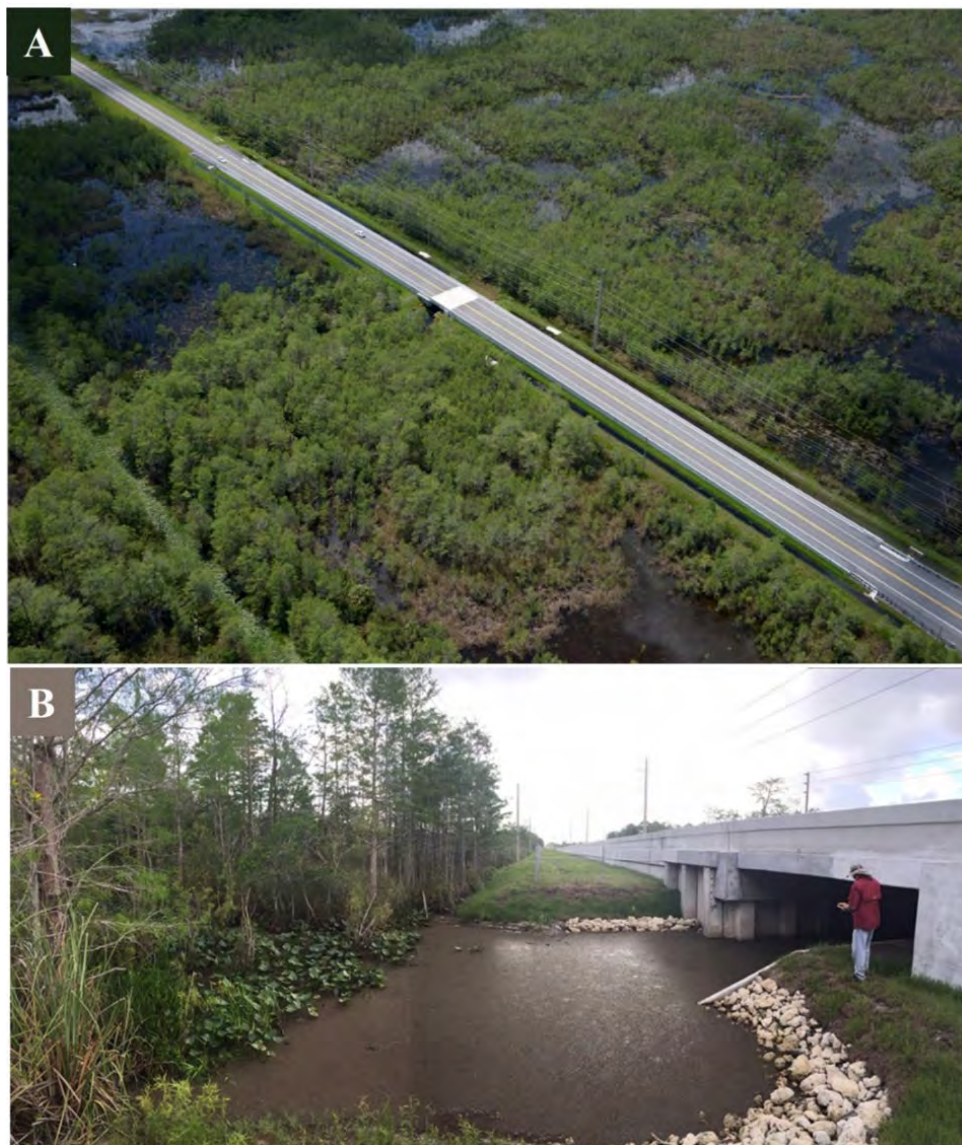
Figure 4.16. (A) Aerial and (B) ground view perspectives of the PGA Blvd. Bridge project. (Photos by FDOT).
