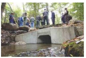
Replacing old pipe culverts with new bottomless, three-sided culverts helps provide passage for fish and other aquatic species. Such projects often necessitate the efforts of multiple partners to accomplish, such as here with Trout Unlimited's involvement with a Gulf Brook culvert in Pepperell, MA. Photo: NRWA Archives.
