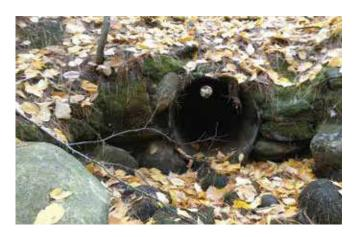
Poorly or undersized culverts can create high water velocity, turbulence, and/or inadequate water depths within the culvert leading to migration barriers for fish and other aquatic species. They also restrict natural stream flows, particularly during floods.
